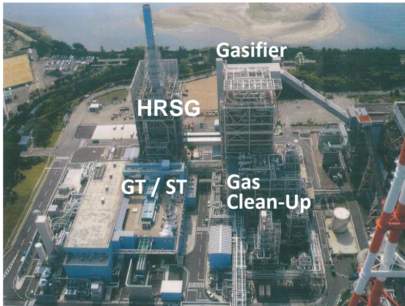
Figure 50. 250 MW IGCC Demonstration Plant 32
