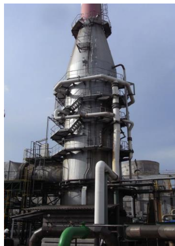
54MW Power Plant in Thailand
