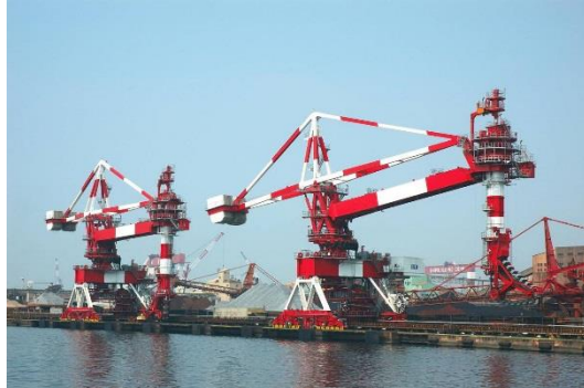
Figure 78. Bucket Elevator Continuous Ship Unloader (CSU) 1
