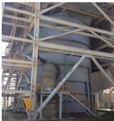
350MW Power Plant in Morocco
