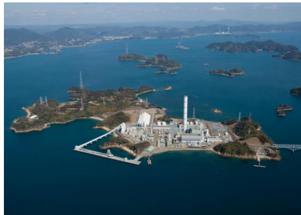
Osaki CoolGen integrated coal gasification fuel cell combined cycle (IGFC) with CO 2 capture demonstration project in Japan
