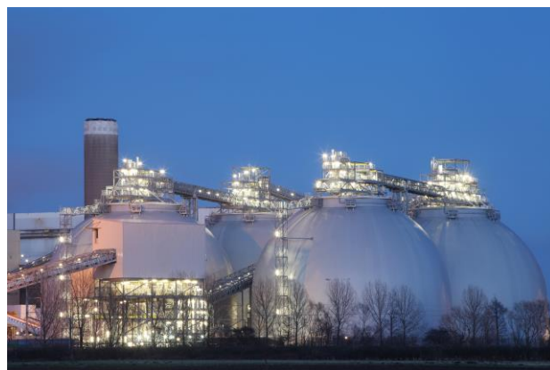
Biomass domes at Drax power plant, Yorkshire, UK
