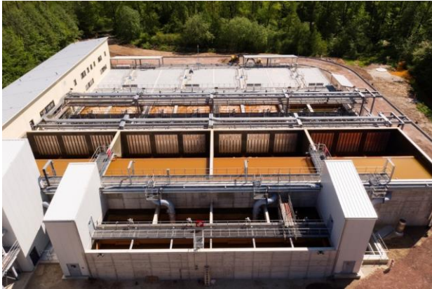
Profen mine-water treatment plant
