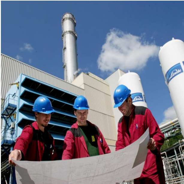
Oxygen separation plant at the Vresová IGCC power plant in the Czech Republic
