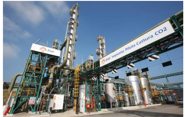
CO 2 capture plant at the 2 600 MW Brindisi Sud coal-fired power plant operated by ENEL in Italy
