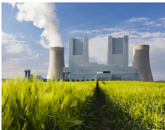
Neurath F&G Power Station, Germany
